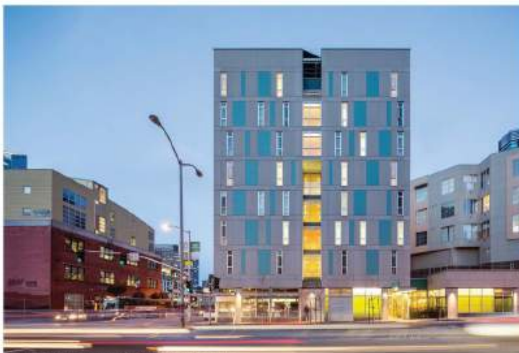
ESSEX STREET FACADE WITH BUILDING ENTRANCE AND CORNER RETAIL
